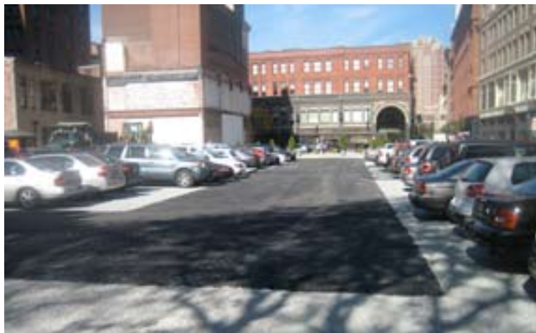
pervious parking spaces encourage stormwater recharge
