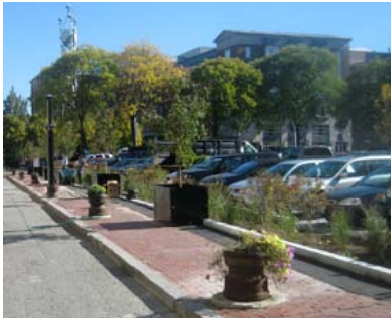
bioretention along the parking edge filters & infiltrates runoff
